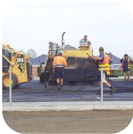
The court under construction at South Colac
