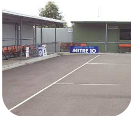
The new facilities at South Colac
